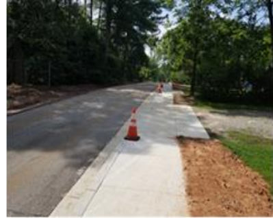
City of Dacula – Infrastructure Improvements; Street
