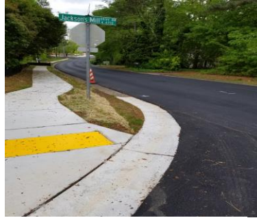
City of Lilburn –ADA sidewalks
